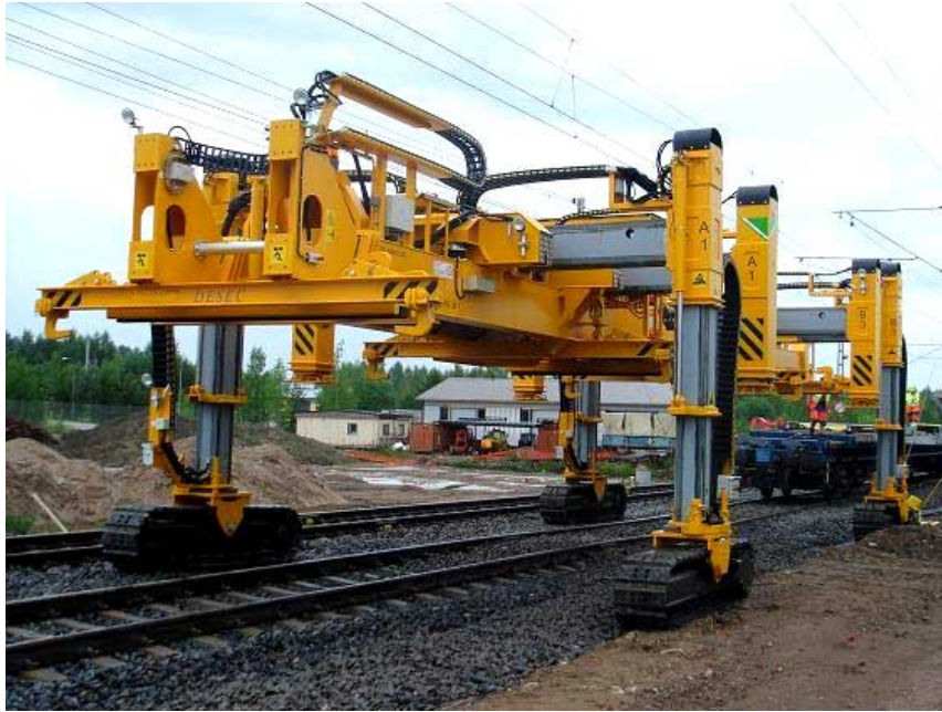
Figure 29: Remtek track laying machine
