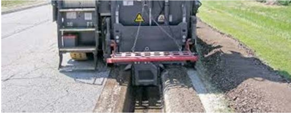
Figure 25: Milling machine forming trench
