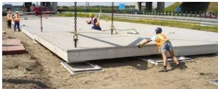
Figure 27: Installation of Modieslab prefabricated section
