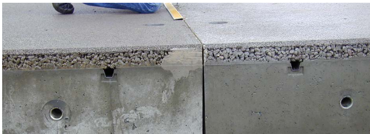
Figure 28: Modieslab sections in-situ
